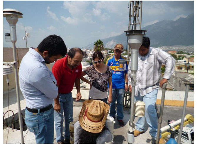
Trainings for local technicians for operation of equipment sampling PM2.5 (small volume) at the monitoring station in Monterrey, Nuevo Leon, during the implementation of measuring activity.
