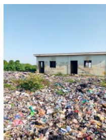
Left: Access road to the final disposal site which was recently cleaned. Middle: Dumping site of the final disposal site. Right: Current situation of the office building constructed by the project (Photographs by the site manager, June 10, 2022)
