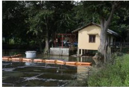
Intake and Pump house
