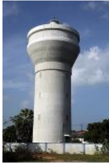
Paranthan Elevated Water Tower
