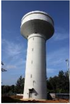
Kilinochchi Elevated Water Tower
