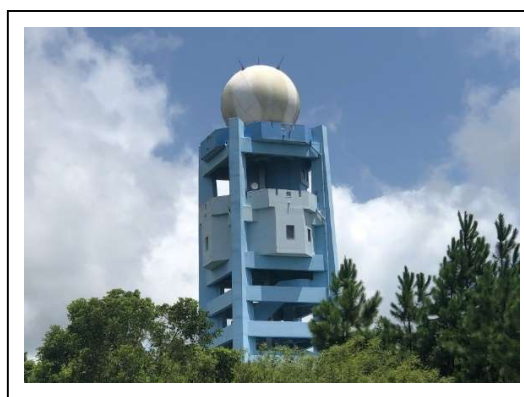
Meteorological radar tower (source: External Evaluator)
