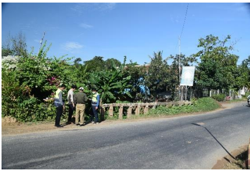
Inspection Ruessei Srok Bridge along NR21B (previously known as NR110, where pilot project was conducted,
