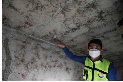
The repairing work is in good condition
