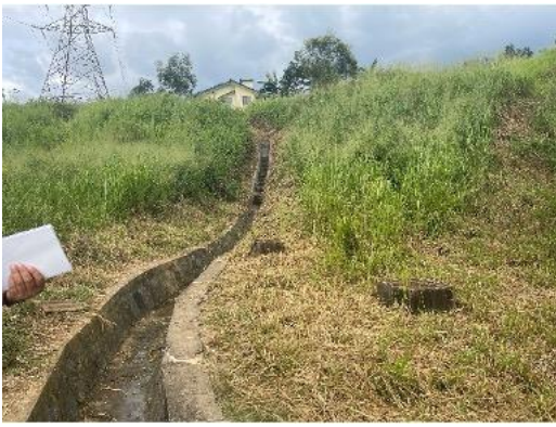
(Drainage in Badulusirigama, Badulla) No damages and function well.
