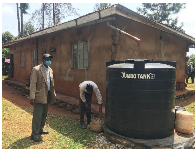
A household implementing rainwater harvesting system to ease reproductive burden on women, Nyeri County
