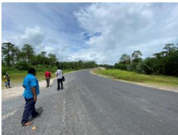
An approach road leading to the Kapiura Bridge has been constructed (Source: External Evaluator)
