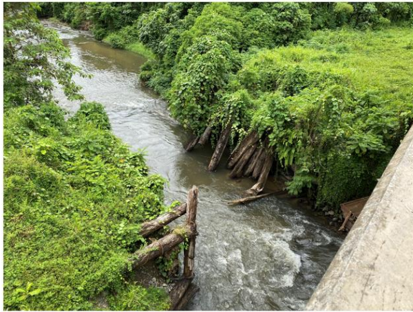
Log bridge incompletely demolished near the Aum Bridge (Source: External Evaluator)
