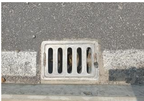
Drainage Outlet of Chuzomsa Bridge
