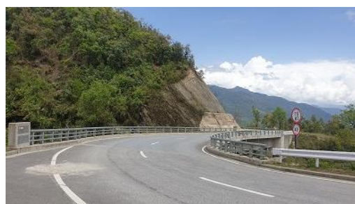
Curving Zalamchu Bridge
