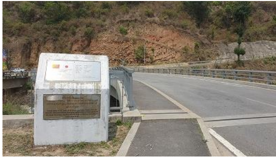
Sidewalk of Chuzomsa Bridge
