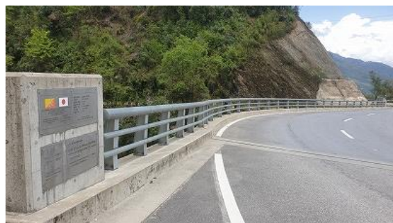
Well-cleaned Zalamchu Bridge
