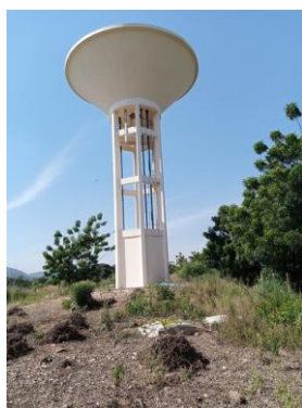
Elevated water tank in Mako in Kédougou Region
