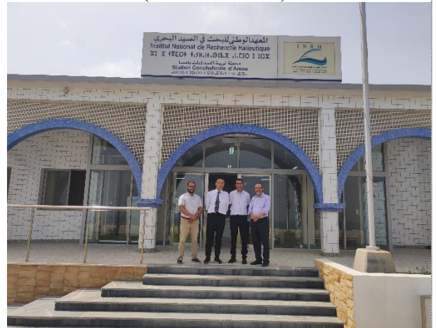
Main entrance of the facility built under the project (source: Evaluator)
