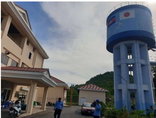
Office Building and Elevated Water Tank
