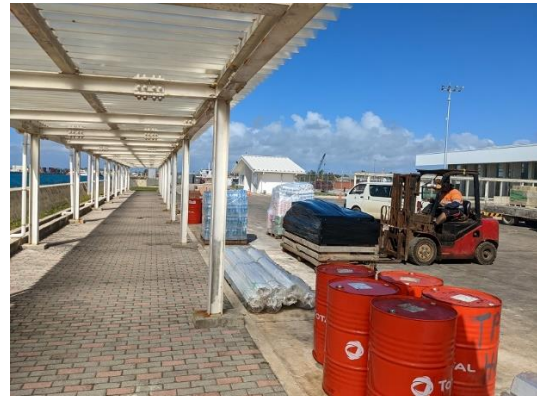
Covered passenger walkway (Photo by External Evaluator)
