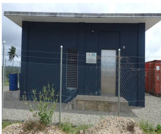
Outside of MW Transmitter House constructed under the project.
