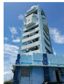
Meteorological radar station
