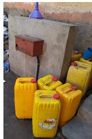
Individual hydrant and a polyethylene container for carrying water (Photo by the evaluator)
