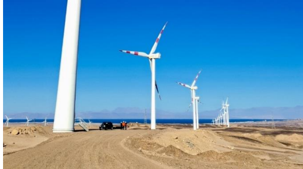
Developed Wind Power Facility (Gulf of El Zayt)
