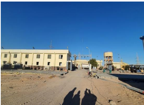
Photo 1: Full View of the Substation (EETC Facility)
