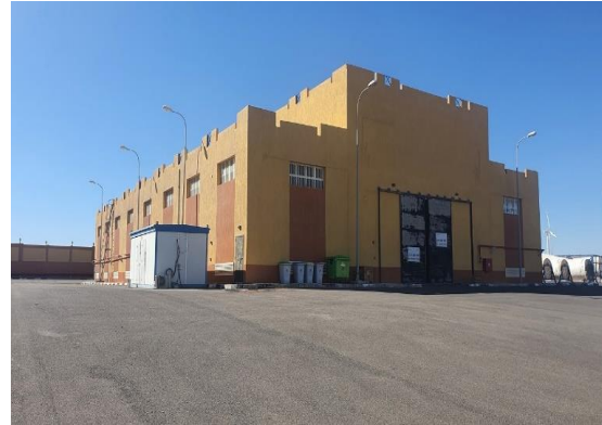
Photo 7: Spare Parts Storage Facility
