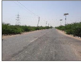
Internal Road of Sanad III Industrial Estate (Khorai Estate)
