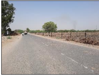
Connecting Road to Sanand II Industrial Estate
