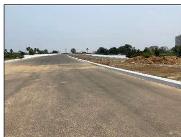
Construction of Bypass Road
