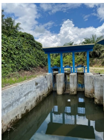
Drainage Canal (Tommo Subproject)
