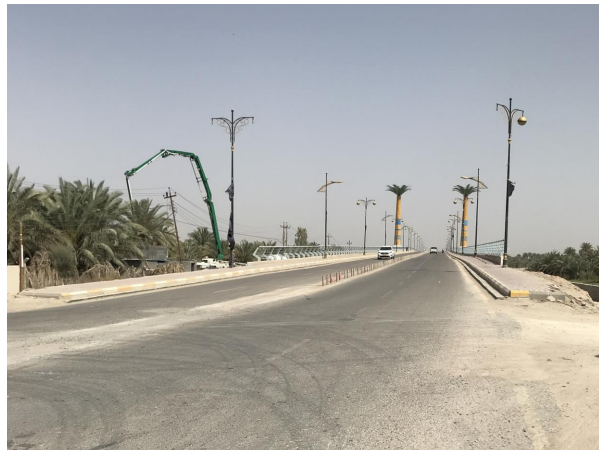
Samawah North Bridge (source: Ex-post evaluation team 1 )
