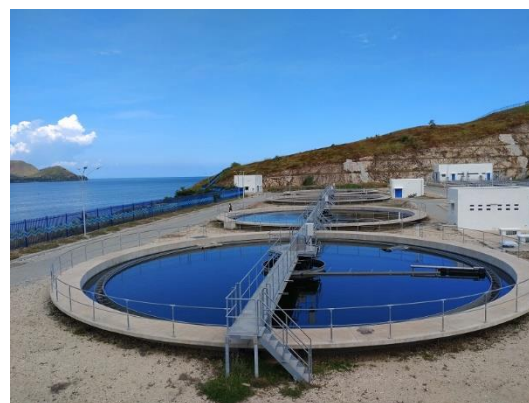
Joyce Bay Sewage Treatment Plant developed under the ODA Loan project (Source: Japan Economic Research Institute)
