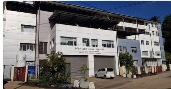
New hospital building at Theldeniya BH
