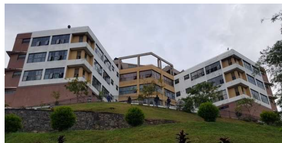
New hospital building at Warakapola BH
