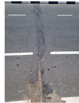
After the repair work
