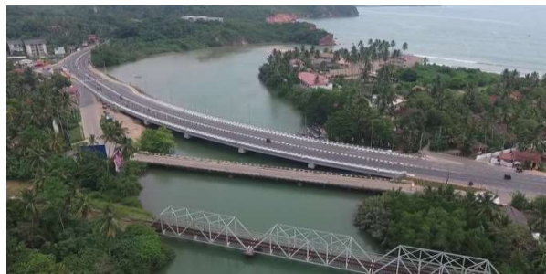
Polwathumodara Bridge, Matara District, Southern Province
