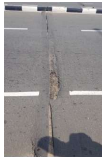
Before the repair work
