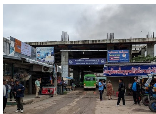
Central Bus Station where construction has been suspended
