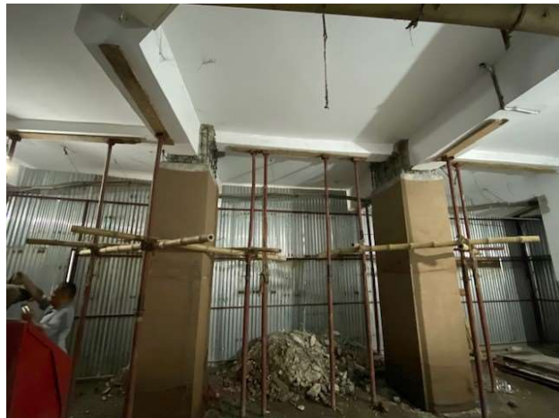
Seismic retrofitting by the implementing agency
