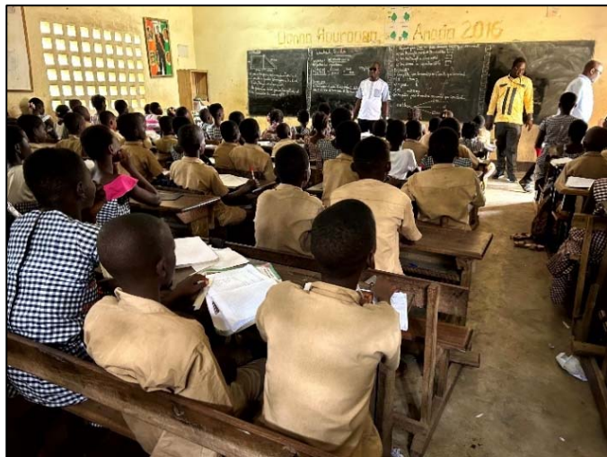
Photo 3 Classroom after School Renovation (Abobo) Source: Photo taken by the evaluator.
