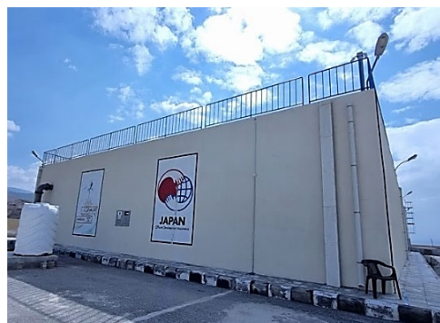
Ma'adi Reservoir (Phase 1)
