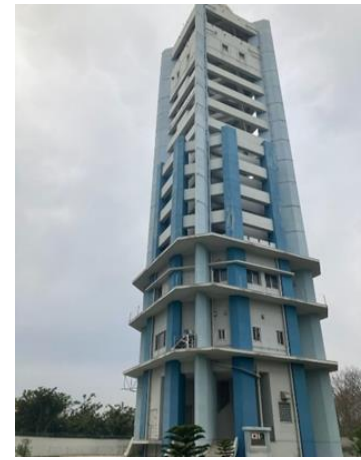
Developed Meteorological Radar Tower (Inside Pakistan Meteorological Department Islamabad Head Office) (Source: picture taken by the evaluator)
