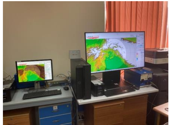
Picture 2: Meteorological Radar Data Display System (PMD Meteorological Office Inside the New Islamabad International Airport) (Source: picture taken by the evaluator)
