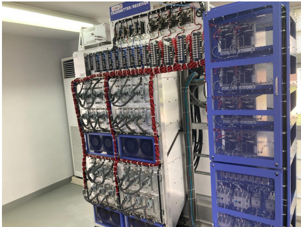
Picture 3: Meteorological Data Trunk Communication System (partial) (PMD Lahore Flood Forecasting Division) (Source: picture taken by the local survey assistant)
