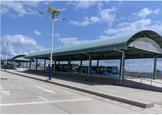
On-going Construction of BRT Phase II in Dar es Salaam
