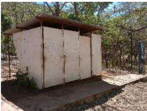
Photo 7. Toilet Booths which Used to be Utilized Before (Madriz)
