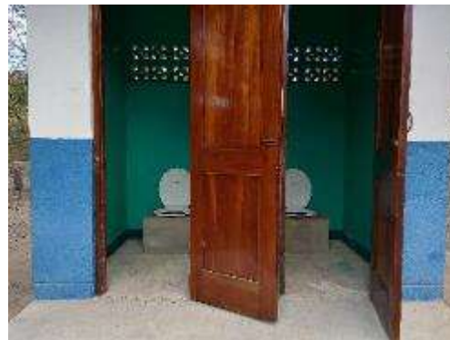
Photo 8. Toilet Booths Constructed by the Project (Nueva Segovia)
