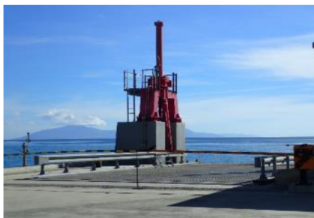
Movable ramp (source: evaluator)
