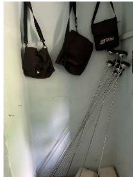
Leak detection equipment at PWD, Curtorim, functional
