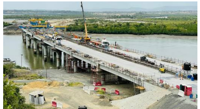
Construction of the Mombasa Southern Bypass Road (ongoing)
