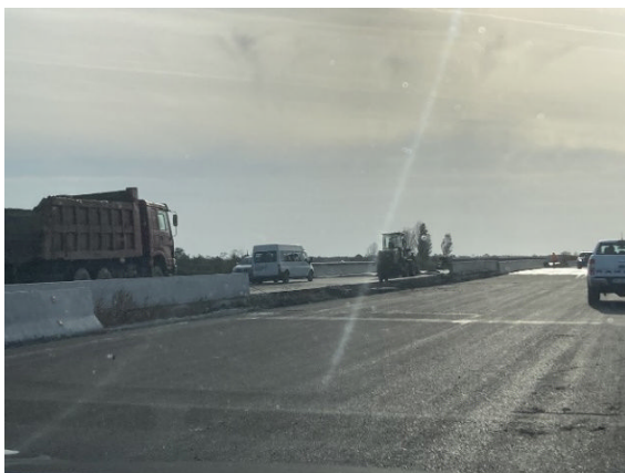
Photograph 3: Road Construction on the West Side of Samtredia
