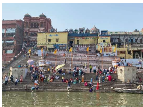
Bathing Ghats along the Ganges River, renovated by the Project
