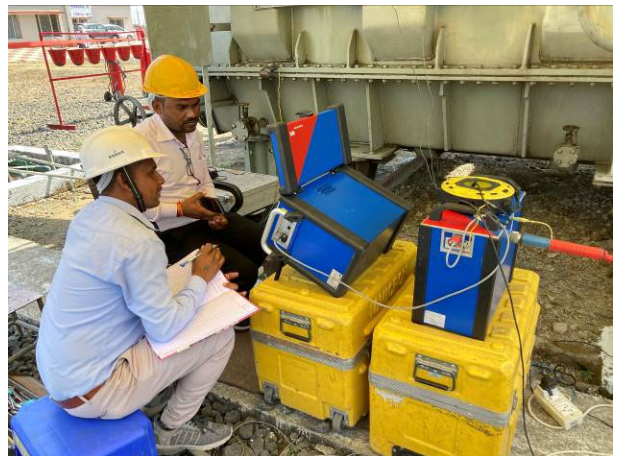
Periodic inspection of transformers (Dhar substation: photo by the external evaluator)
