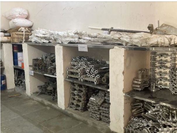
Stock of spare parts at substation (Gorabazar substation: photo by the external evaluator)
