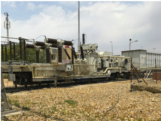
Mobile substation
