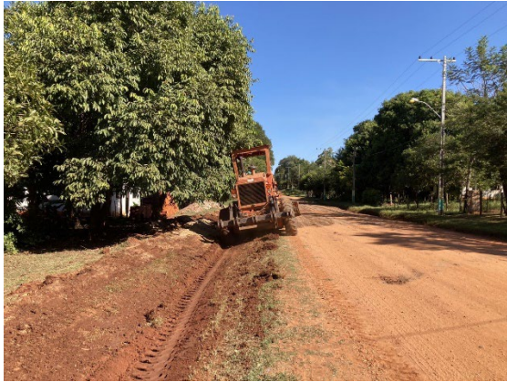
Maintenance work by MOPC
