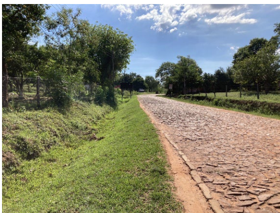
Rubble paved section
