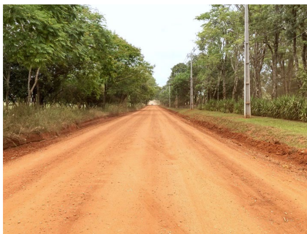
Gravel paved rural road 1
