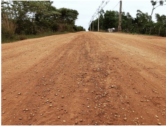
Gravel paved section
