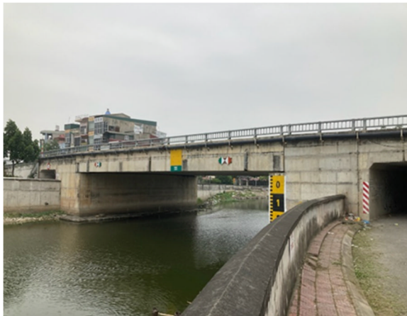
Picture 3: Cat Bridge (Hai Duong Province) (Source: Photographed by the evaluator)
