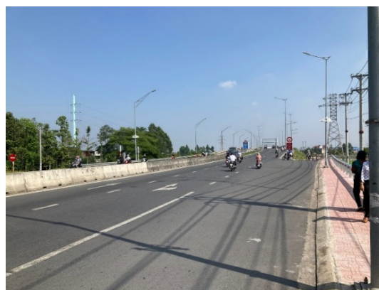
Tan An Bridge (Long An Province) (Source: Photographed by the evaluator)
