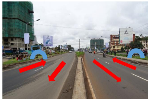
Photo 2: Upon completion, Ngong Road has two lanes instead of one, with drainage ditches on both sides and sidewalks separated from the road. (Source Project Completion Report)
