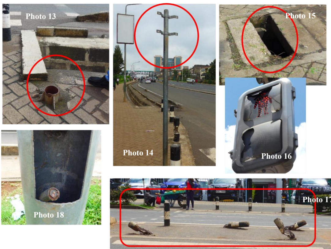
(Clockwise from top left) Photo 13: A road sign cut off at the base, Photo 14: A stolen sign, Photo 15: A stolen drain cover, Photo 16: A destroyed traffic light, Photo 17: A knocked-down concrete pole, Photo 18: A cut and stolen street light cable (Photo by the external evaluator)
