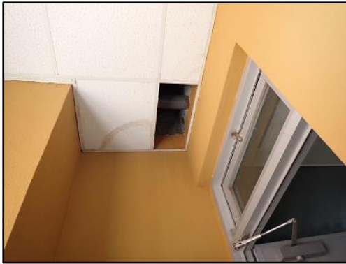
Photo 5: Leakage areas identified during the first on-site survey (confirmed repairment during the second survey) (source: taken by the evaluator)
