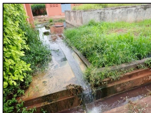
Photo 4: Wastewater Flowing out of a Septic Tank (source: taken by the evaluator)
