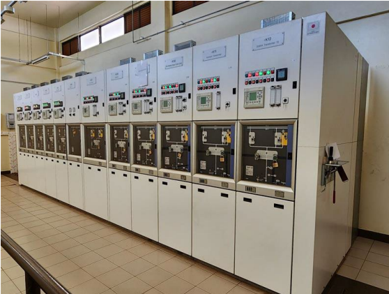
Picture 1: Ndear Substation 15kV Switchgear panel (Source: picture taken by the external evaluator)
