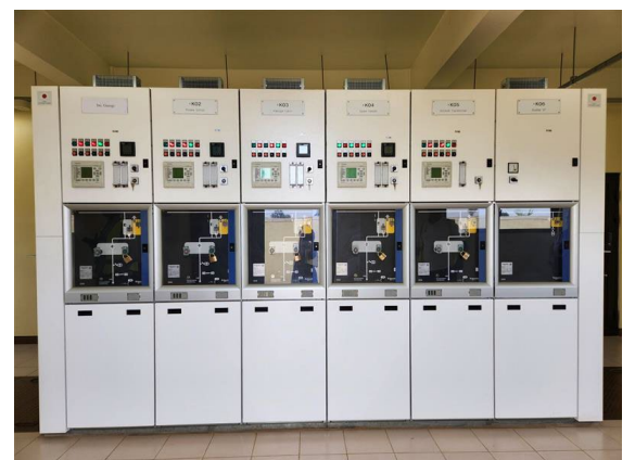
Picture 6: Kabuga RMU Switching Station 15 kV Switchgear Panel (Source: picture taken by the external evaluator)
