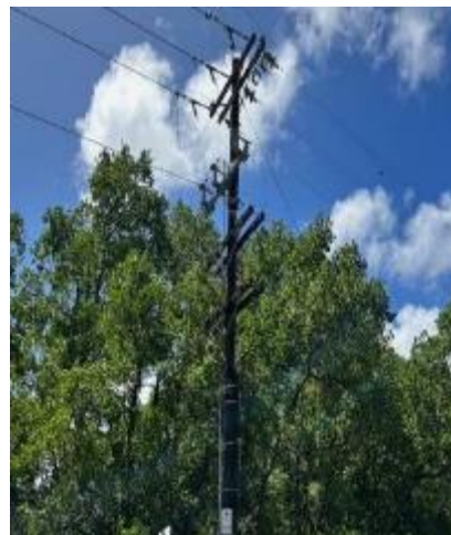
Photo 2: Underground cable connection pole (Source: External evaluator)
