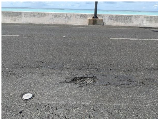
Photo 5: Pothole on the Nippon Causeway (Source: Photo taken by the external evaluator)
