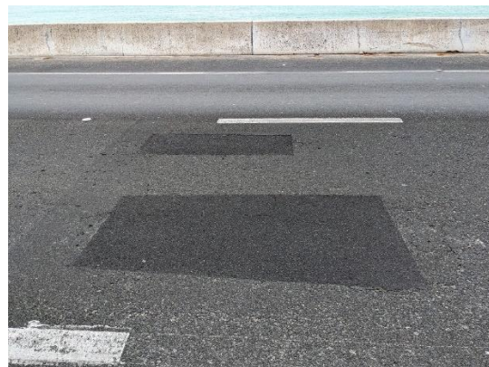
Photo 6: Road surface repaired by MISE (Source: Photo taken by the external evaluator)
