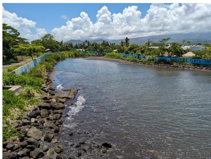
Photo 2: Revetment along the Vaisigano River (Source: Photo taken by the External Evaluator)
