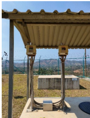
Flow meter (photographed by the evaluator)
