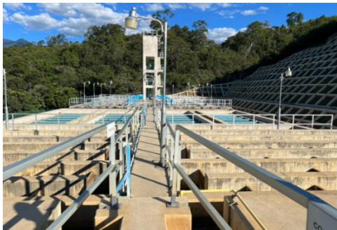
Sedimentation pond and filtration pond (photographed by the evaluator)
