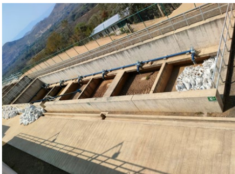
Sludge drying bed (photographed by the evaluator)
