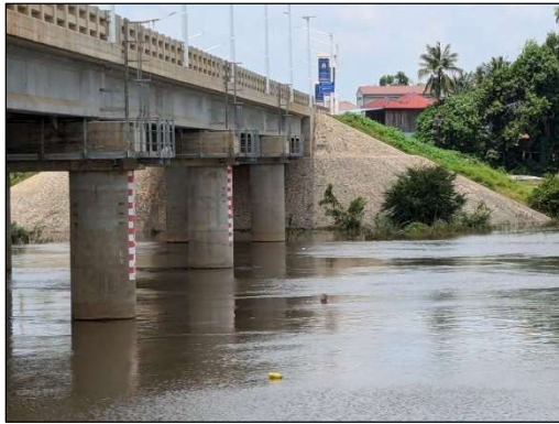
Photo 5: Height markings to bridge girders (Peam Te Bridge) (Source: Evaluator's photo)
