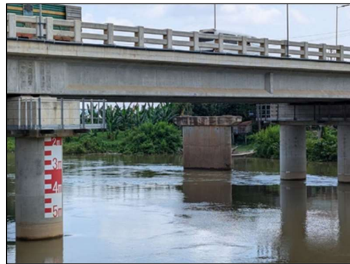
Photo 6: Height markings to bridge girders (Prek Chhloung Bridge) (Source: Evaluator's photo)
