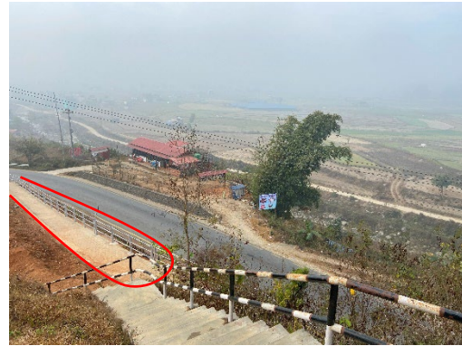
Photo (9) Newly constructed sidewalk (red line)
