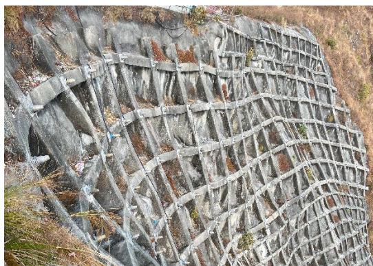
Photo (2) Anchor construction of Sta. 17+400
