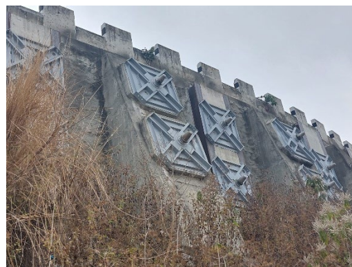
Photo (3) Anchor construction of Sta.33+440
