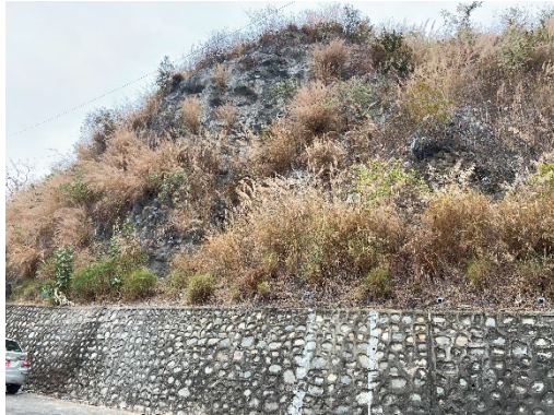
Photo (6) Anchor construction of Sta.15+520
