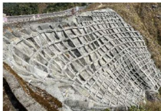
Photo (1) Anchor works developed by the project 1
