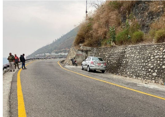
Photo (7) Road condition of Sta.15+520
