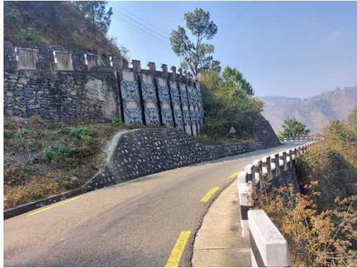
Photo (4) Anchor construction of Sta.33+695
