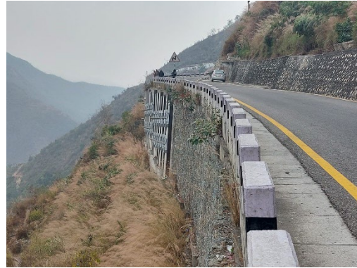
Photo (5) Anchor construction of Sta.11+620
