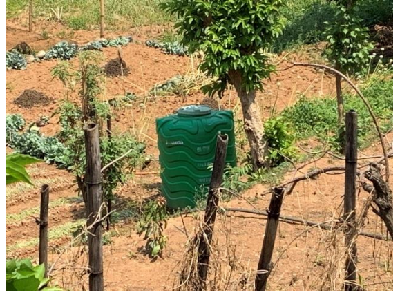
Irrigation reservoir/pipe Roshi Rural Municipality, Kavre District
